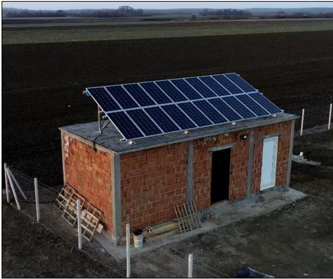
Fig. 2. Front side of the considered PV generator (the source of this photograph is https://tkpenergy.com/portfolio-items/pozarevac-solarna-elektrana-i-navodnjavnje-35ha-plantaza-tresanja/ ).
