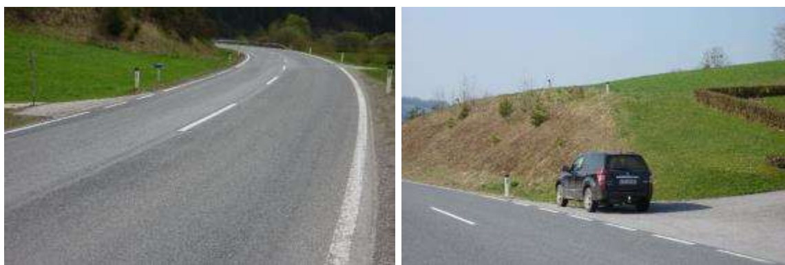
Fig. 2 – Devices on guide posts a) B 124 km 27.8, b) L 576 km 1.7
