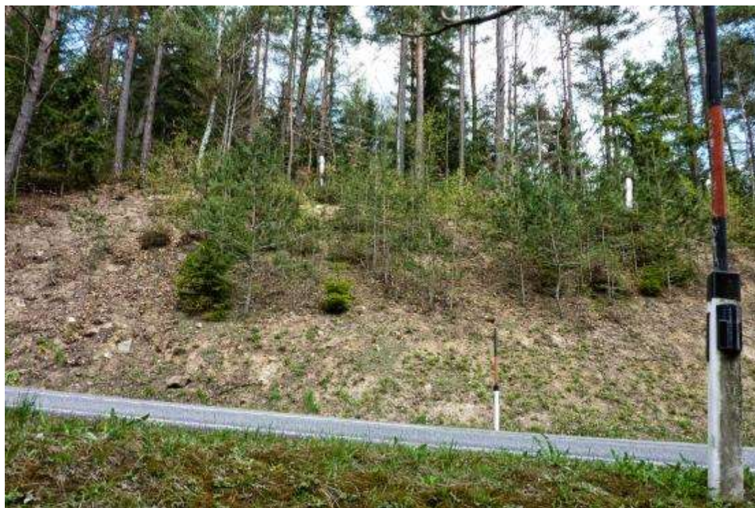
Fig. 1 – Devices beside the road and on topological shoulders mounted on guide posts
